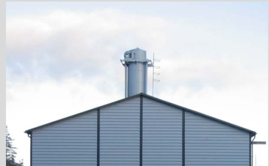
Top of MVR falling film evaporator.
